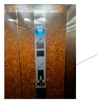
The arrow is pointing to the yellow button on the COP which is the Alarm Sounder. If the Alarm Sounder is pressed/held it will enable the passenger(s) trapped inside the lift to call for emergency help.
